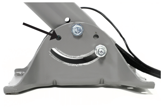
Figure 2: Wrong (footplate, large-hole side)
